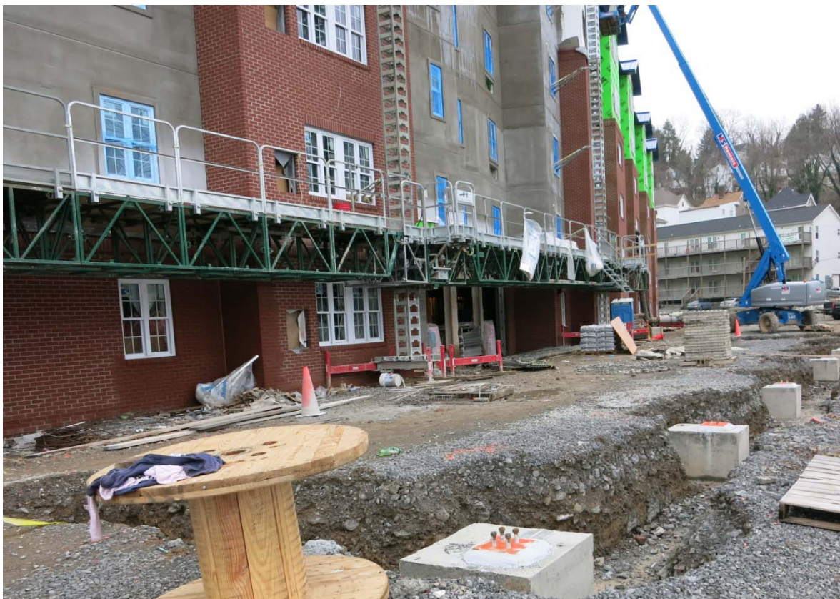
Stucco installation on Central Place Apartments (background), Harless Center Footings (foreground)
